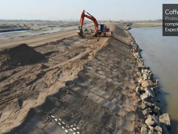
Coffer Dam Protected With Stone, 50% complete Expected Completion: Jun 30, 2024
